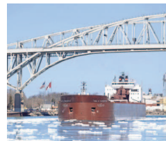
A freighter passes under the Blue Water Bridge near Port Huron. MARK R. BUMMEL/TIMES HERALD
